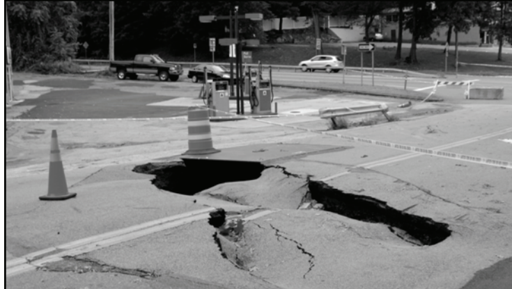
Collapsed Roadway between Route 9A and Pleasantville Road
