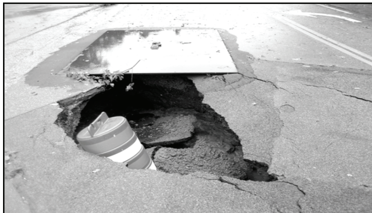
Collapsed Roadway between Route 9A and Pleasantville Road
