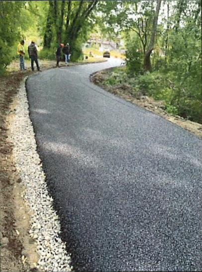
**1050 PLEASANTVILLE ROAD PARKING LOT** Following the demolition of the Wells Fargo Bank, DPW staff performed all the parking lot modifications. Working involving installing belgian block curb stones, drainage, signage, line striping, electrical site lighting and pavement replacement.
