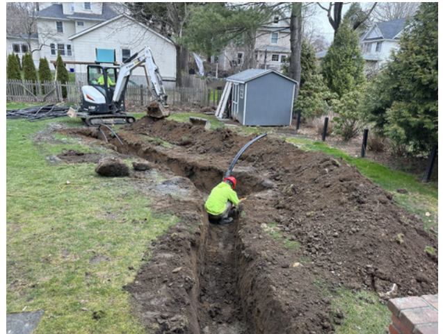
Trenching from boreholes to the foundation
